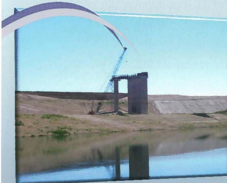
At the bottom of the tower, the concrete walls are eight feet thick to compensate for the earth load as well as the pressure of the water that would be placed on the walls of the tower if the reservoir were full.
