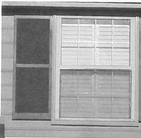
Right: Windows with original, correctly-sized shutters.
