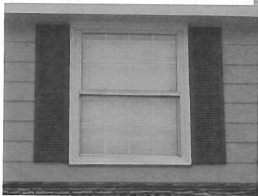
Left: Window with incorrectly-sized shutters.
